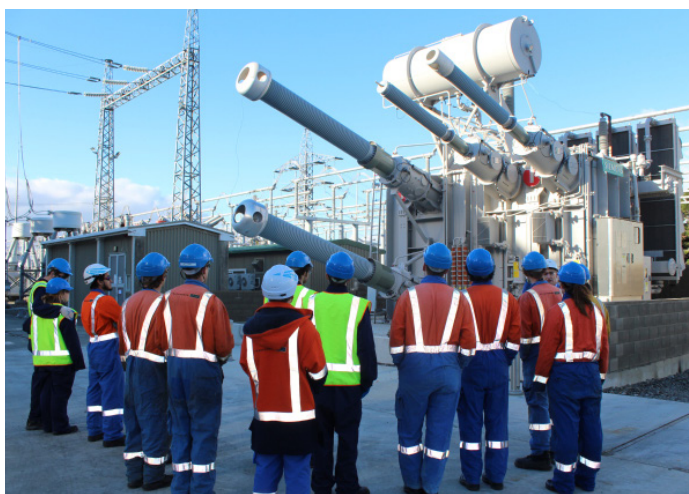
Students at Haywards Substation during a multi-day field trip
